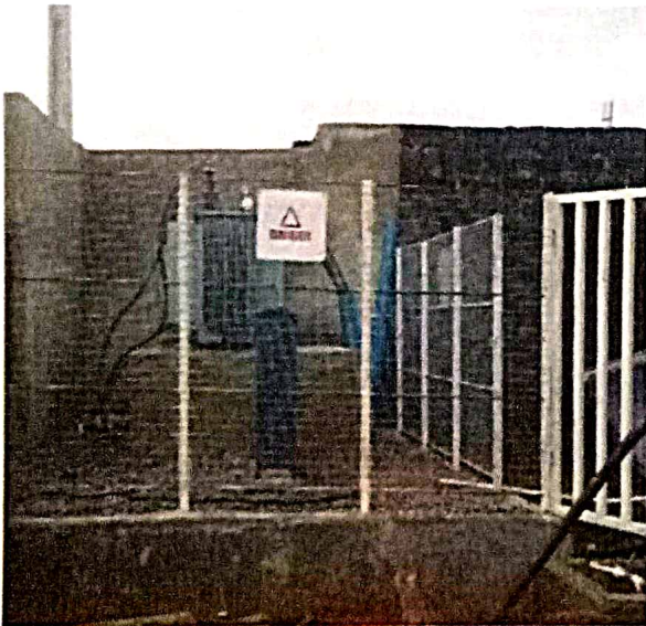
A newly constructed standard substation with danger sign, standard fencing, graveling.
