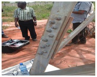
i. order In to prevent easy climbing access by vandals, all the step bolts below the anticlimbing devices should be removed from position as advised ii. All tower location within visible erosion prone areas along the entire The following were also observed;
