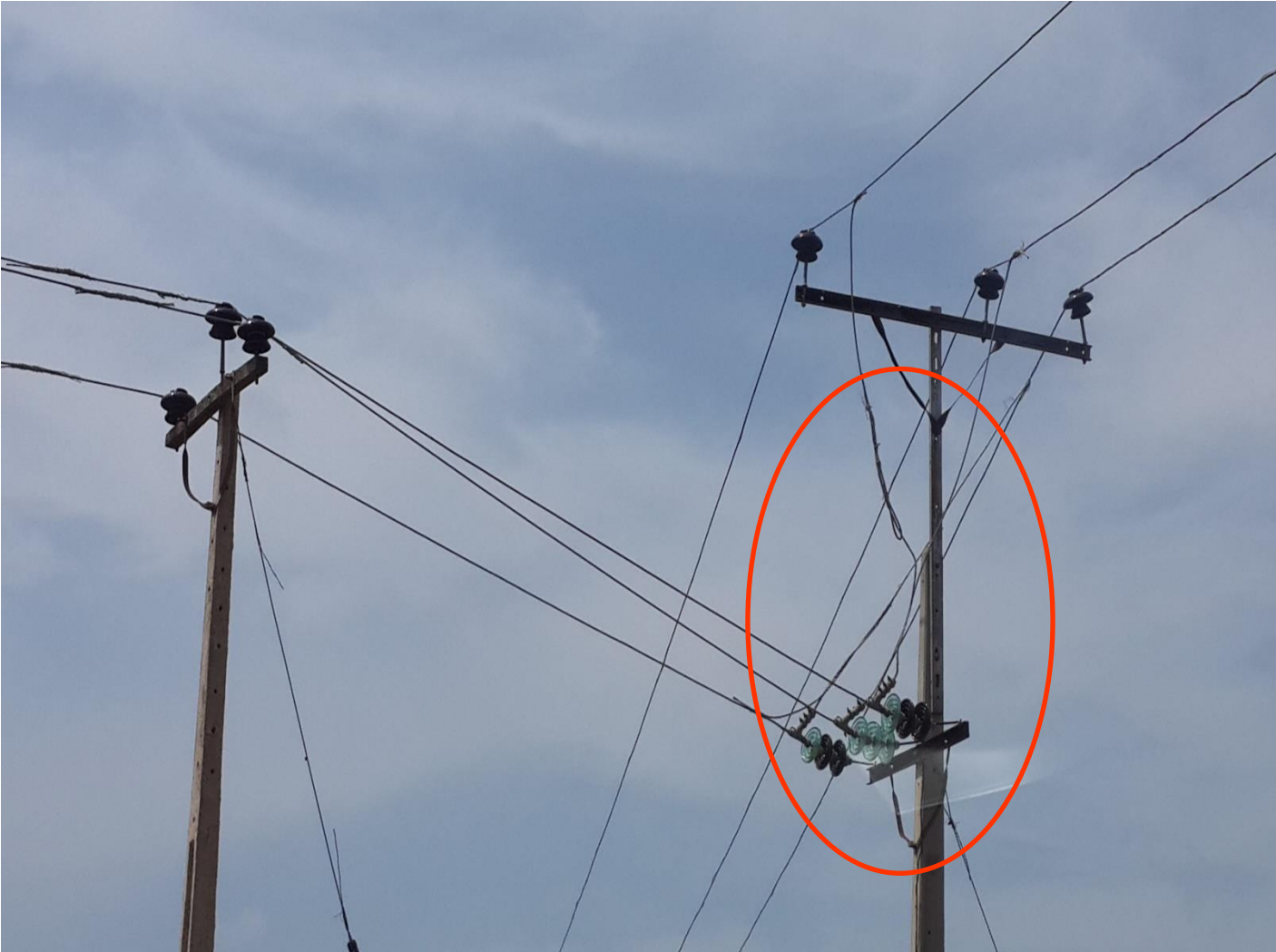
Poor terminations and dangerous Tees-off at Kuje and Jabi, Abuja FCT
