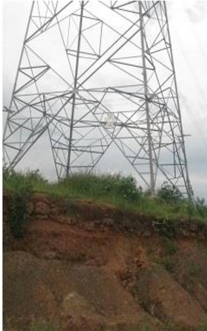
River Bank erosion and reported sand dredging activities in Otamiri, Imo State, and Amechi village, Enugu State, endangering transmission line towers.
