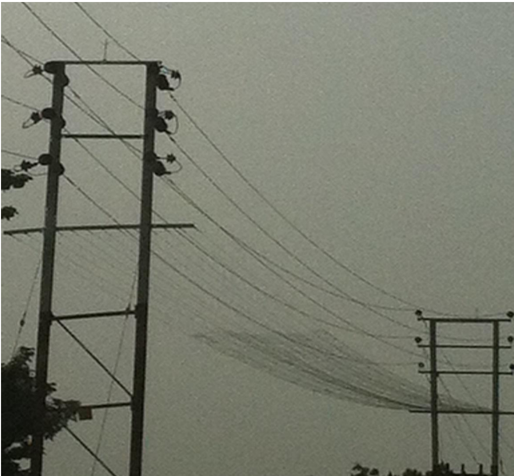
Cradle Guards installed over bridge /expressway crossings in Wuse Zone 4, and Wuse II, Abuja, FCT
