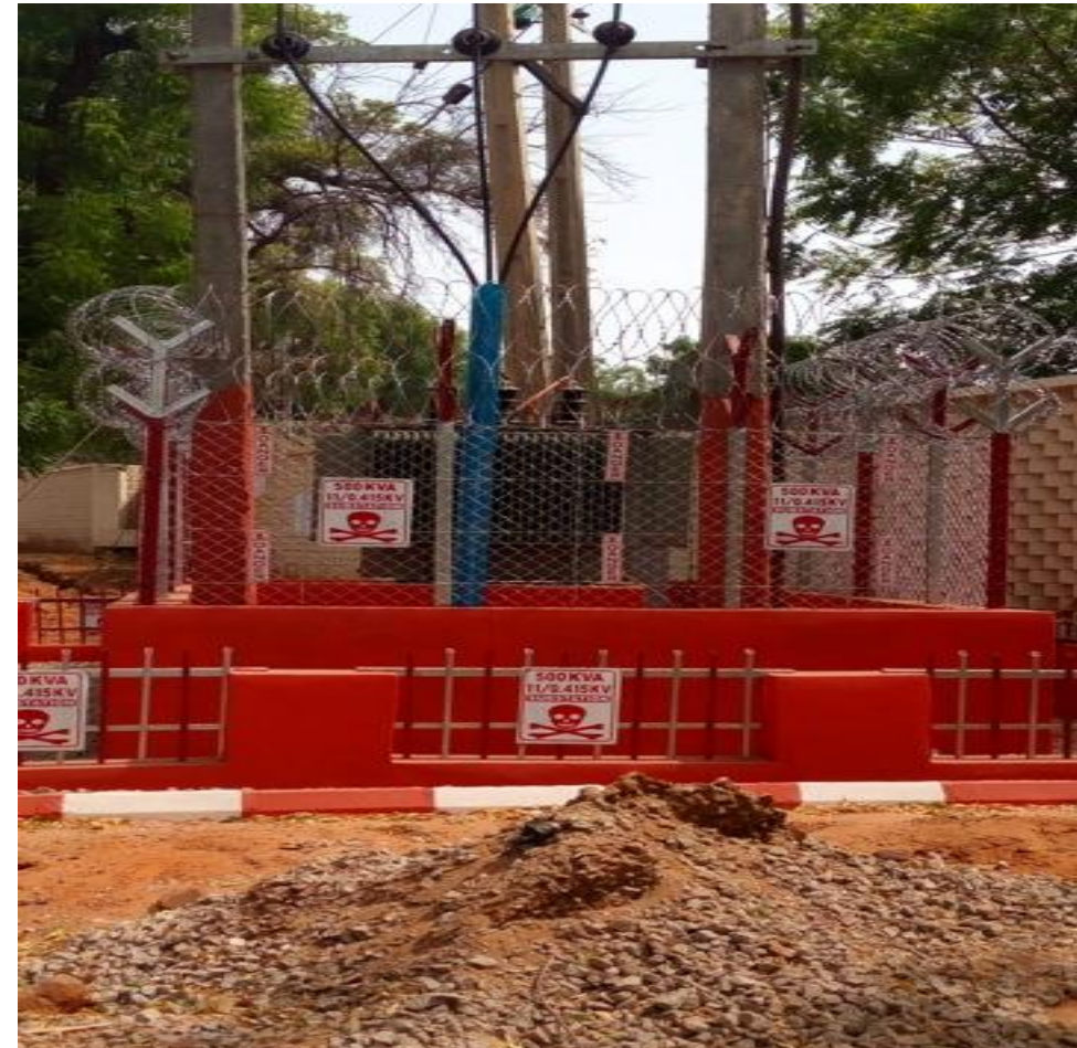
A well designed and constructed substation in GRA, Sokoto.
