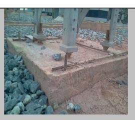
The overall weighy of the gantry structure can tilt the affected gantries out of balance thereby resulting in major construction defects.
