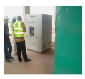
The installed 3.15MVA11/0.415KV, transformer was not properly protected with either wire mesh (as was the case for the 500Kva, 11/0.415kV distribution transformer and the
