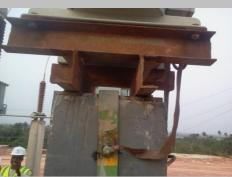
Use of galvanized bolts and nuts and galvanized steel channels is recommended.
