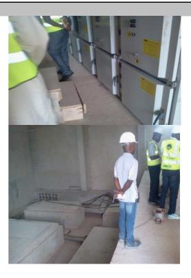
Provision of recommended safety measures would secure both lives and installed infrastrucure. The worker captured in the pictorial above can easily slip over into the ditch behind him, hence the need for adequate barriers/rails to guard possible slippage.
