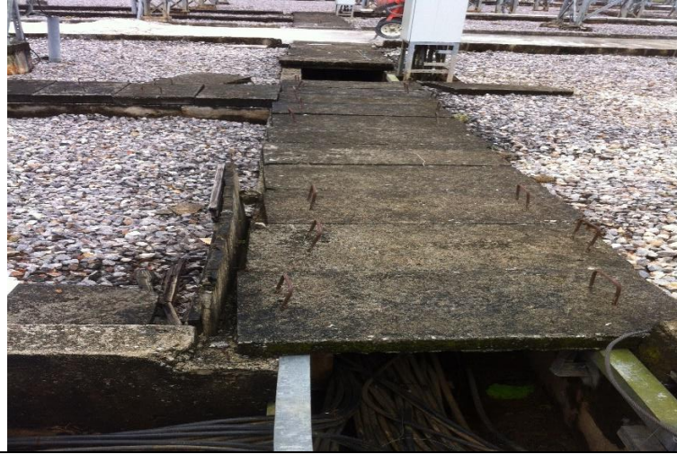
Exposed cable trenches
