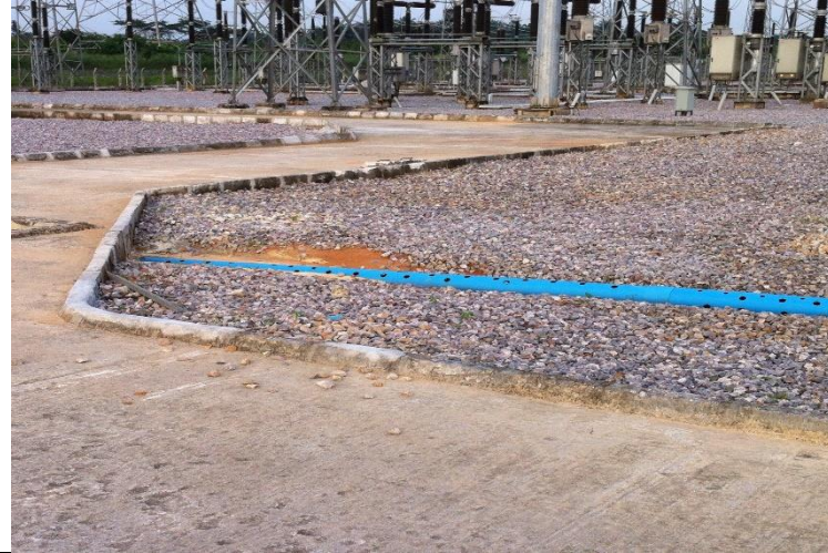
Exposed cable trenches
