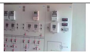
of the ix. Some labelling on the control panel are not explicit enough. On some panels the label upper indicates Jos 2- Jos 1 whilst the line diagram below indicates Jos 1- Jos 2
