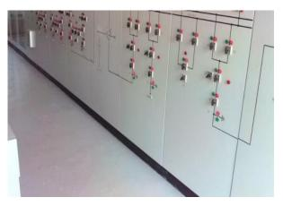
The control panel indicators should also be re-wired to indicate RED when the units are ON and green when the units are OFF
