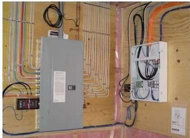
Figure 6: Surface Wiring System
