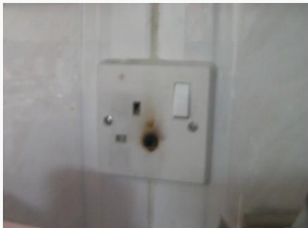
Figure 11: Damaged Socket Outlet
