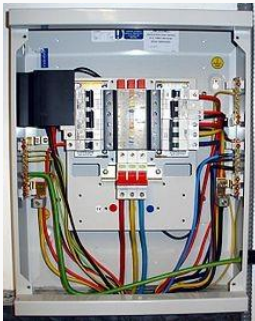
Figure 2: Distribution board
