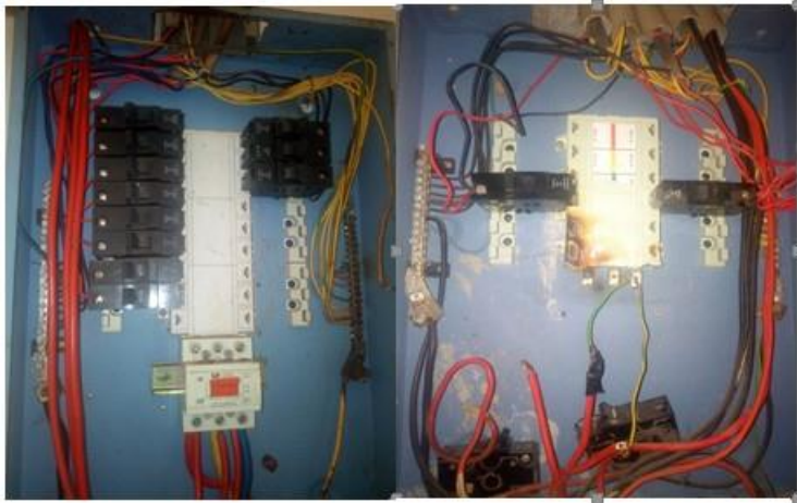
Figure 14: Poor Termination of cables in distribution board
